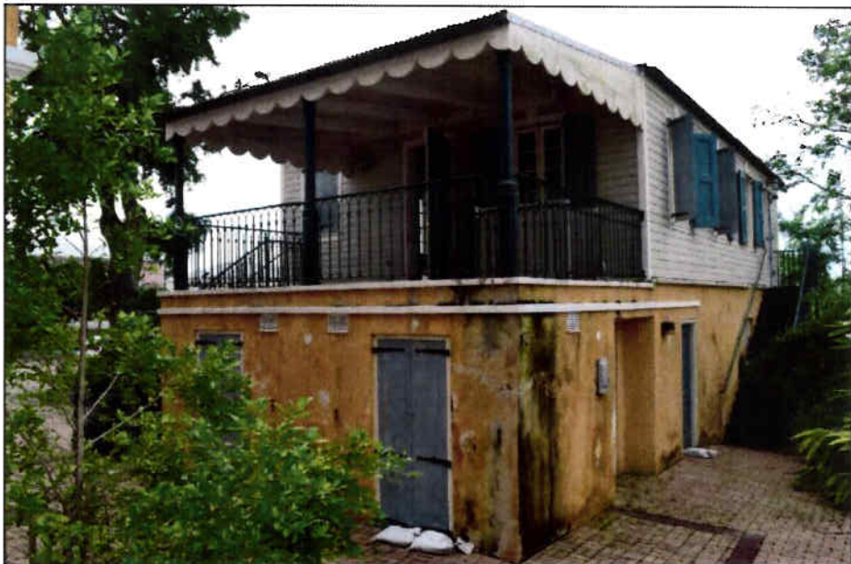
Figure 4: Danish School Kitchen Building, East and North Elevations, Looking Southwest. Taken 11/7/2017.
