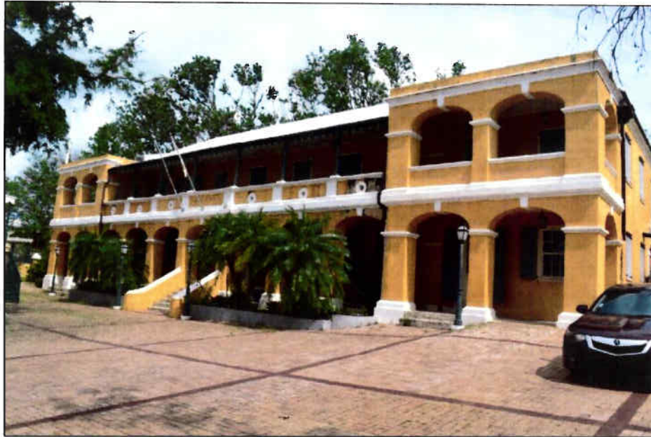
Figure 1: Danish School, Front (West) Elevation, Looking Northeast. Taken 11/7/2017.
