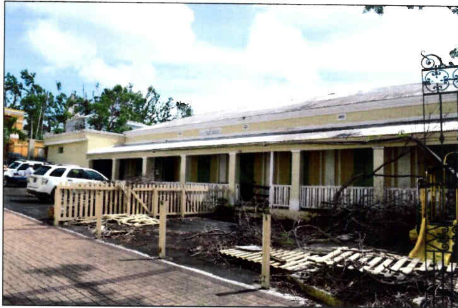
Figure 5: Annex Building, North Elevation, Looking Southeast. Taken 11/7/2017.
