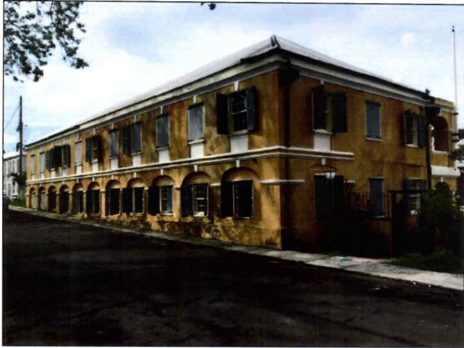
Figure 2: Danish School, Rear (East) and Side (North) Elevations, Looking Southwest. Taken 11/7/2017.
