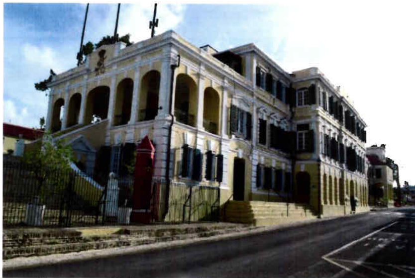
Figure 2: Stucco finish on rubble masonry walls, keystone, pediment, quoins, 1st floor gallery with arched openings, parapet on roof, brick steps, marble busts on stair newel posts, porch gallery with arched openings, plaster pilasters, Danish regent's crest.
