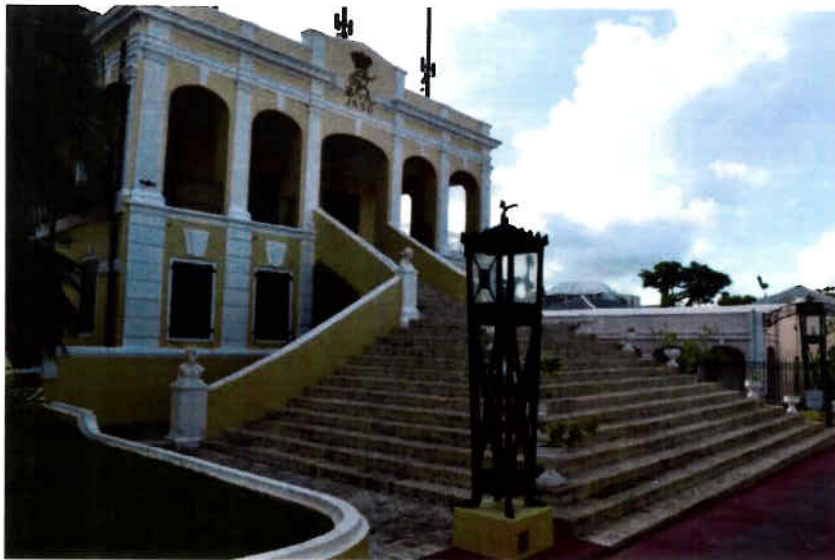
Figure 3: Pilasters, brick steps, marble busts on stair newel posts, arched gallery, plaster pilasters, quoins, Danish regent's crest
