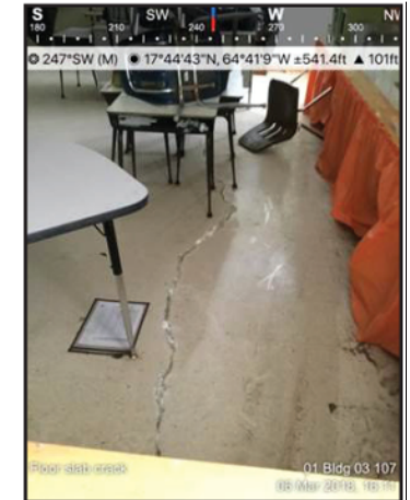
Structural Floor Slab Cracking
