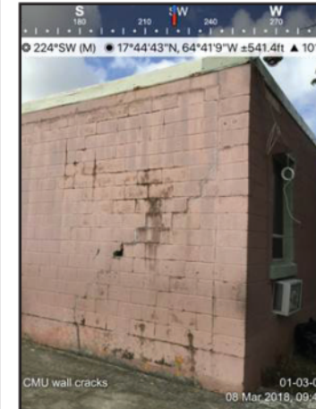
Structural CMU Cracking
