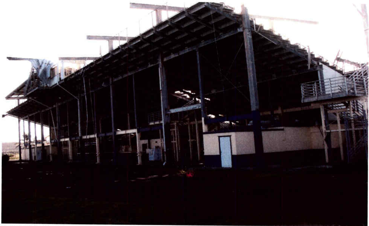
PHOTOS SHOWING THE DAMAGED ROOF
