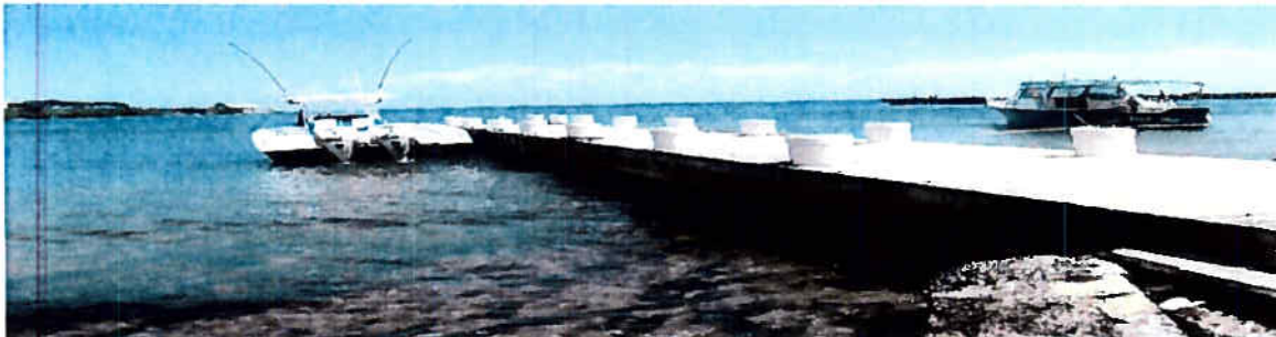
Repairs to the Gallow's Bay Boat Access Dock
