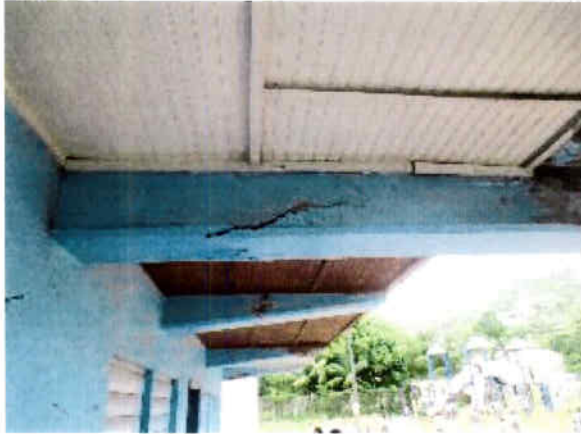
Ulla Muller ES : Cracks in reinforced concrete beam and elevated walkway at Bldg 5.
