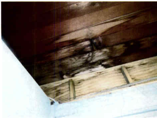
Addelita Cancryn JHS : Leaking at change of material, especially at covered walkways.
