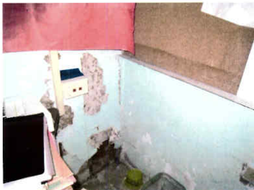
Ricardo Richards ES : hole in the wall from leaks.
