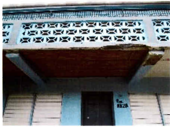
Ulla Muller ES : Cracks in reinforced concrete beam and elevated walkway at Bldg 5.
