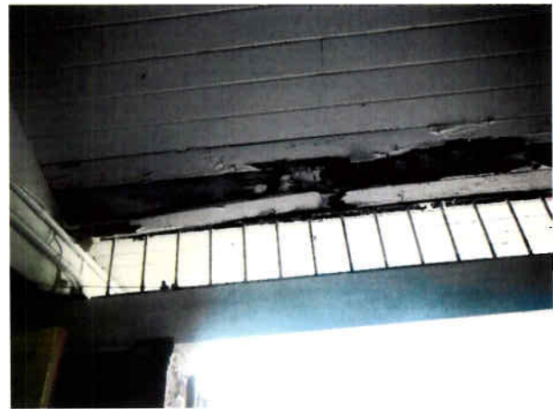
Addelita Cancryn JHS : Leaking at change of material, especially at covered walkways.
