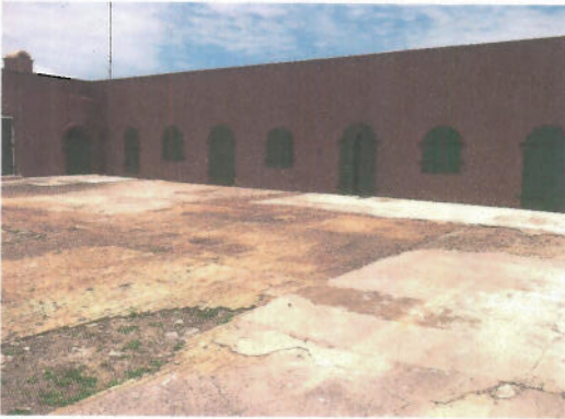
Court Yard looking South-west corner
