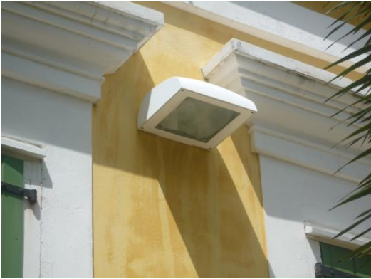
Item No. 01 metal door to be replaced
