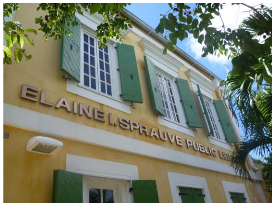
Building's West Side
