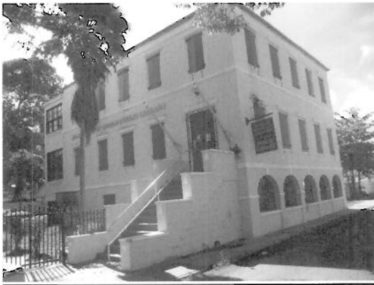
Building's North-west Corner
