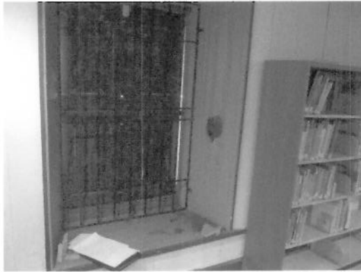
Item No. 36 Repairs around doors and window sill
