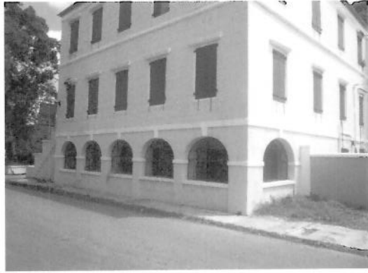
Item No. 3 South-west corner
