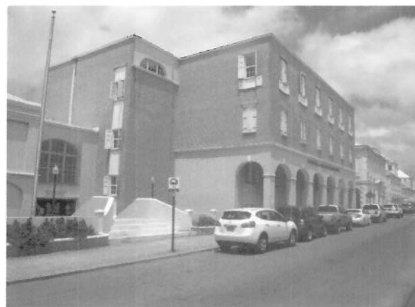
South-West corner view of the Facility
