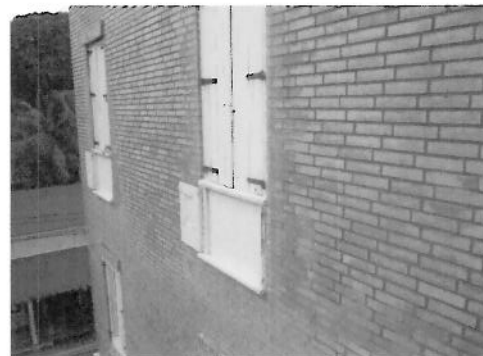
Building's east brick wall
