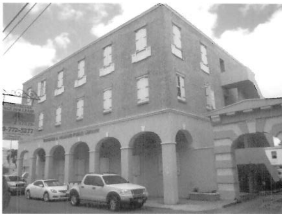
South-East corner view of the Facility
